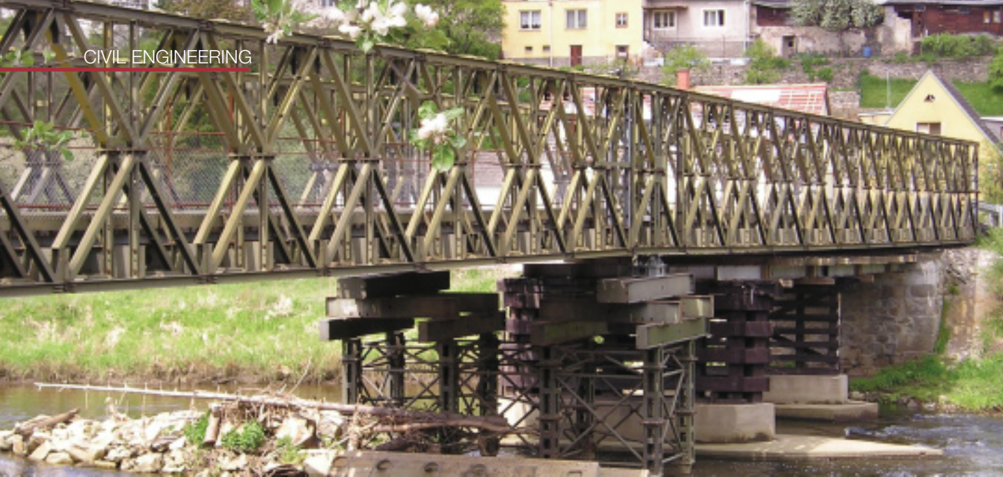
Typical TMS temporary bridge structure in use after a flood
